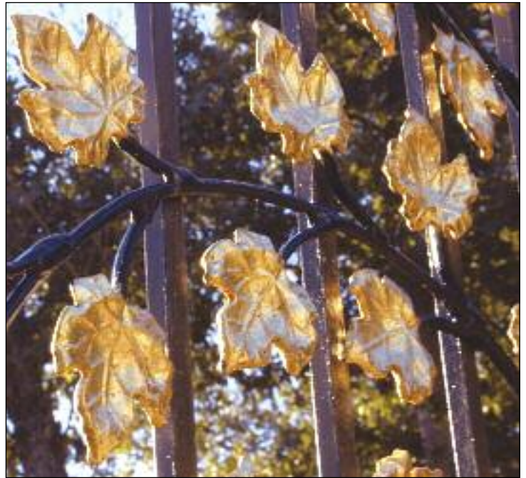
This "gateway of gold," an entry in the 2007 Top Job competition, was fabricated by MH Engineering. German gold leaf (23 \frac{3}{4} -carat) was applied front and back to each of the steel leaves using the traditional oil gilding techniques that have been in use for centuries.
